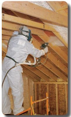
calculating the HVAC load, we normally see numbers from 800-1400 square feet per ton with spray foam insulation vs. 400-600 with conventional insulation.
